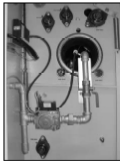
Figure 5.3: IS Series Gas Heat Detail
